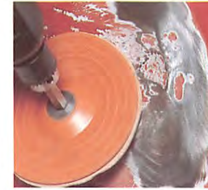
Use a drill and disc or flap wheel to sand down to bare metal for about 1 in. (25 mm) in and around the dent.
