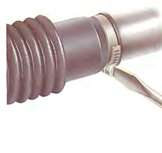
Tighten the clip firmly, but not too much.
