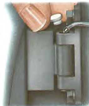
Take the cap off a hollow hinge and fill the pin with heavy oil.
