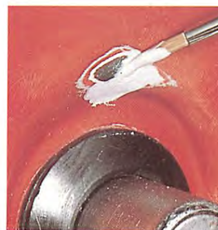
Apply a rust-resistant primer with a small paint brush.
