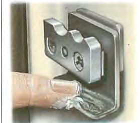
Smear a little petroleum jelly on the metal-to-metal parts of the door latch.
