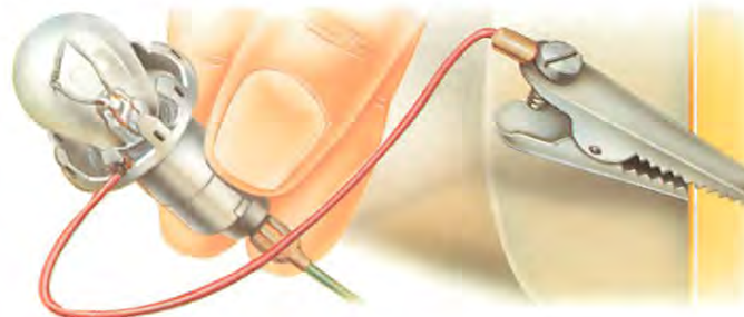
Test a bulb holder by connecting a test lead from the holder to earth, and operating the switch.
