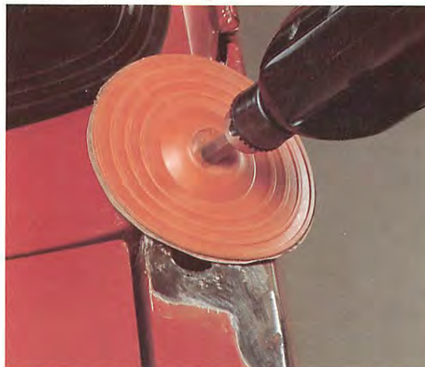
Use an electric drill fitted with a sanding disc or a flap wheel to cut away the surface rust. Take care not to go through good metal.
