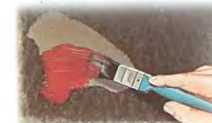
Applying primer to the bare metal gives added protection. Allow it to dry.
