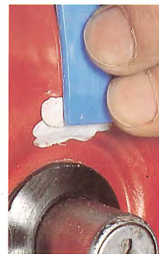
When the primer is dry, use cellulose stopper to bring the area up to the level of the surrounding paintwork.
