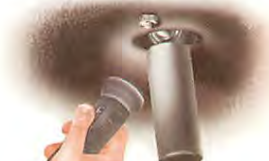
Use a torch to inspect an upper pin-type mounting beneath a domed turret on the wheel arch.
